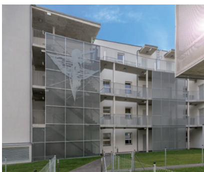
"The Nest": Cladding on the façade and stairwell of Mondscheinweg 2+4, 2130 Mistelbach, designed by artist Carlos Perez, © Irene Schanda
